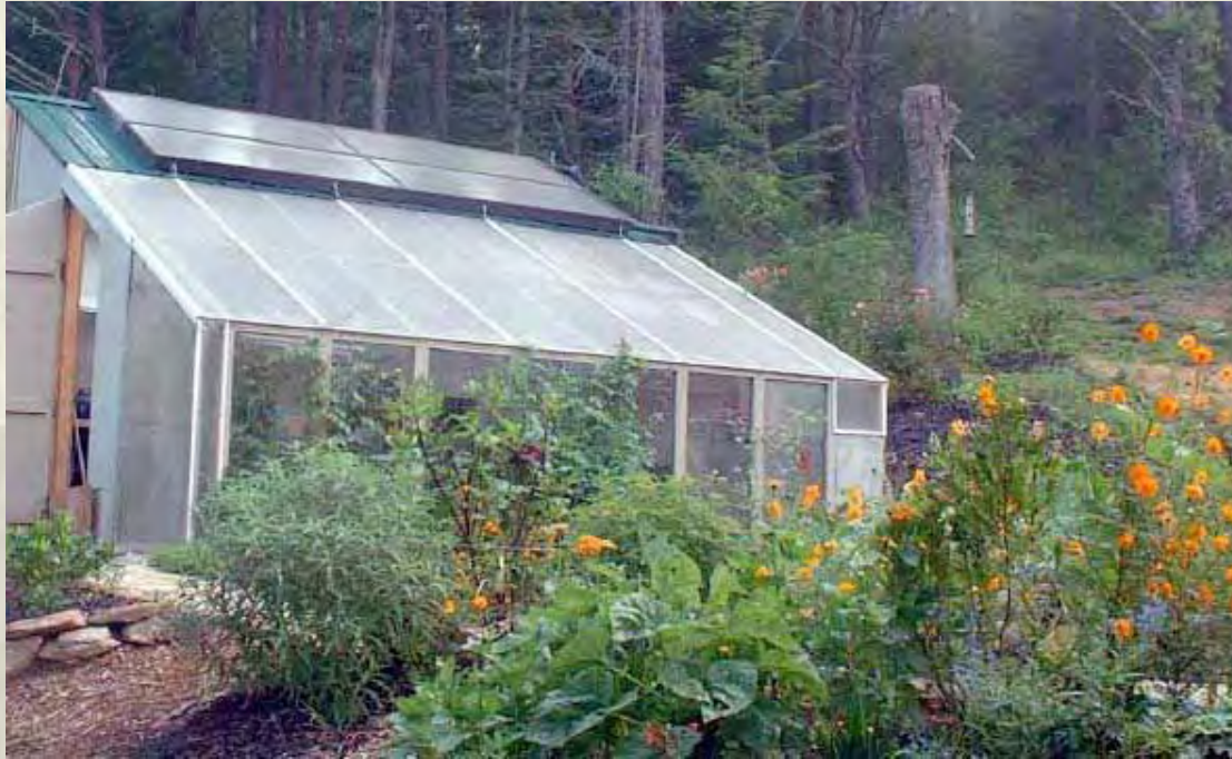
Greenhouse with PV Panels
